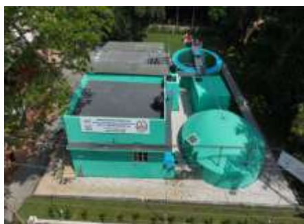
360 KLD STP at General Hospital, Thrissur
