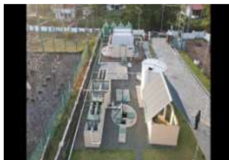
1 MLD CSTP at Padanappalam, Kannur
